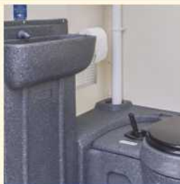
Toilet wash area
