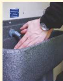
Delivery of hot water
